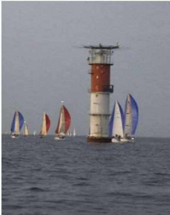
The Helsinki Lighthouse (Finnish: Helsingin majakka; also known as Helsingin kasuuni [2] — Swedish: Helsingfors fyra; Helsingfors kassun) is a caisson-type lighthouse located in the Gulf of Finland, 22 kilometres (12 nautical miles) south of Helsinki's western harbour.
